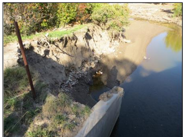
C-16-AF over Buckingham Ditch - Scour at downstream left abutment
