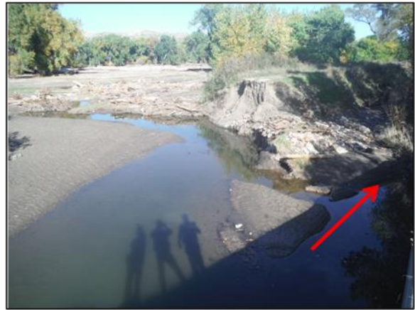
C-16-AF over Buckingham Ditch – The ditch berm or levee was washed out from Big Thompson overtopping
