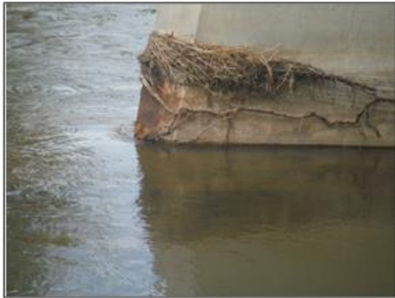
D-16-DA over Boulder Creek – Pier caps exposed beneath water surface
