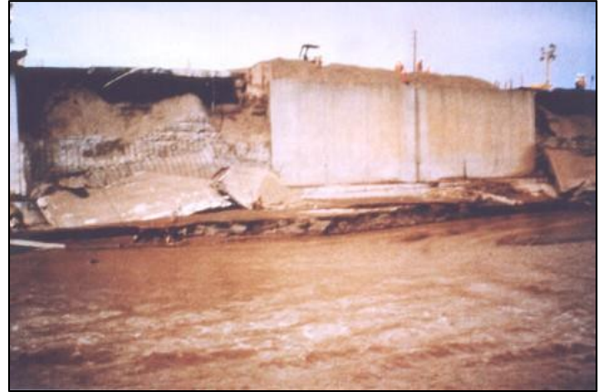
Figure 3. View of the failed bridge from the channel facing downstream. Note the failed left abutment.
