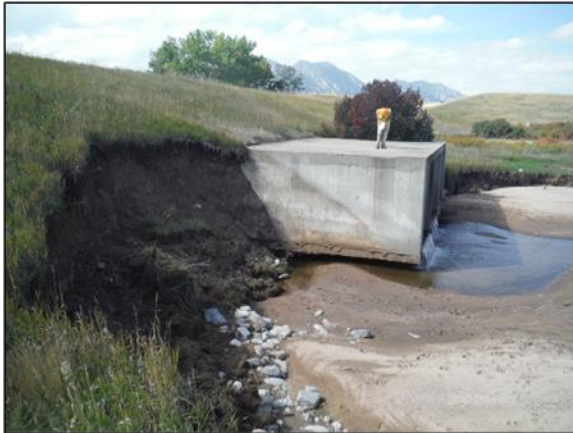
E-16-HB over Coal Creek - Scour at downstream right abutment
