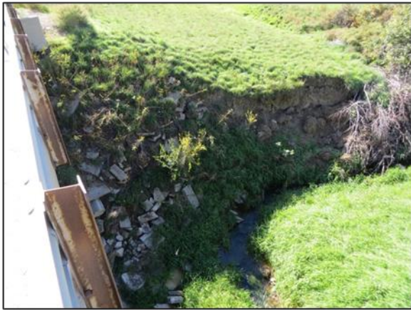
C-17-CZ over Draw – Bank scour on approach to right abutment
