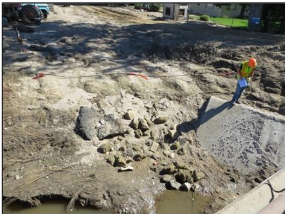
C-17-Z over Big Thompson River - Scour of right emnamkment downstream
