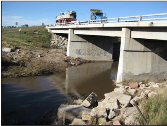
C-17-N over Little Thompson River – Scour at left embankment and downcutting between piers
