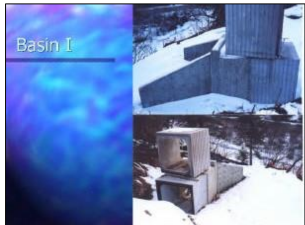
Figure 9. Culvert outlet and pre-fabricated culvert sections
