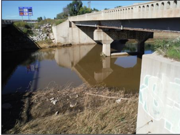
C-17-BL over Big Thompson River – Channel widening and downcutting through bridge section
