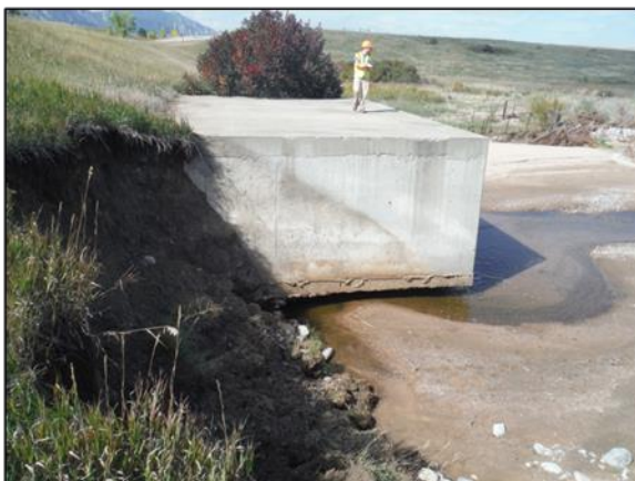
E-16-HB over Coal Creek – Downstream right abutment scour and undermining of structure
