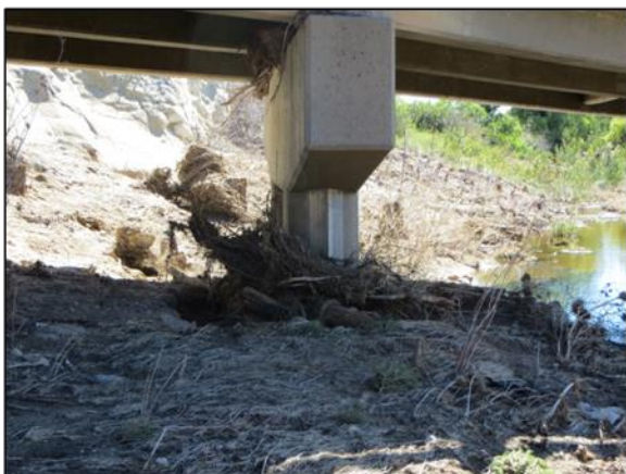
A-17-AC over Lone Tree Creek – Debris accumulation at pier
