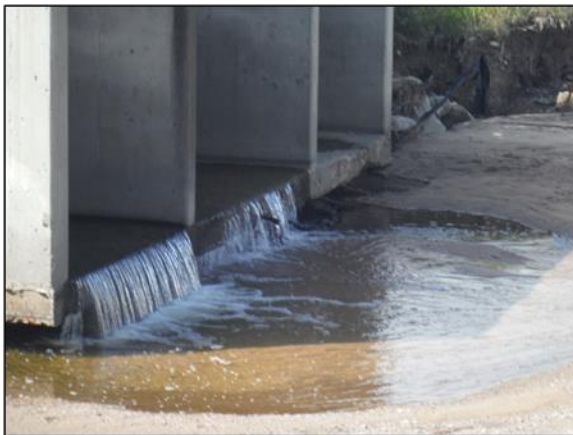
E-16-HB over Coal Creek - Scour at bridge outlet
