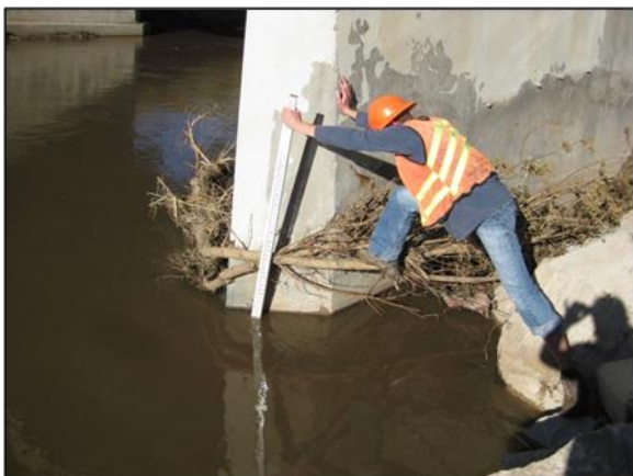
C-17-N over Little Thompson River – Exposed pier cap due to channel degradation and scour
