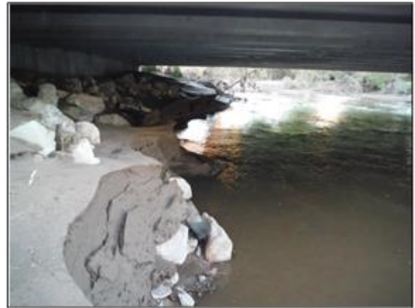
C-16-DK over Little Thompson River – Scour at right abutment
