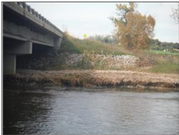
D-16-DA over Boulder Creek – Scouring of channel bank
