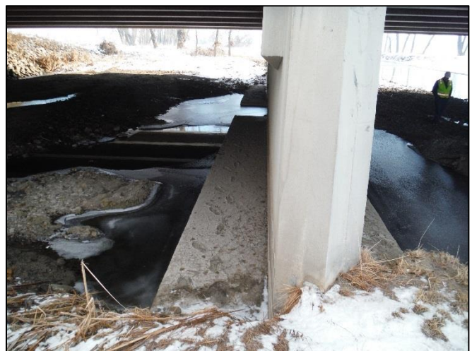
Boulder Creek at US 287, pier scour at spread footers
