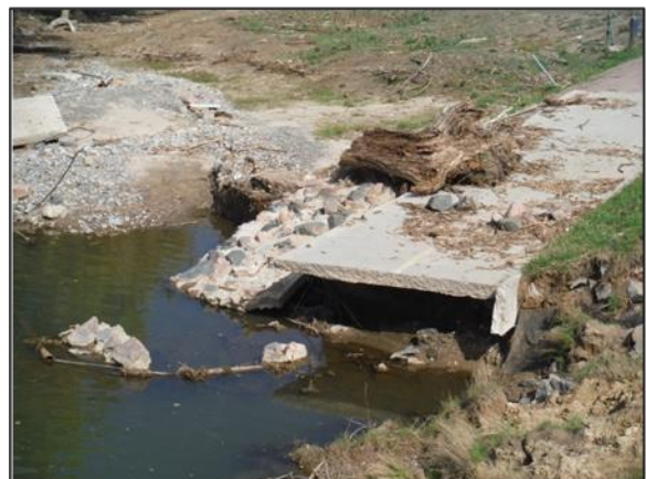
E-16-BC over Coal Creek – Scour damage to adjoining bike path
