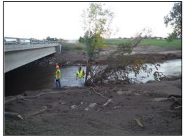
C-16-DK over Little Thompson River – Downstream channel scouring
