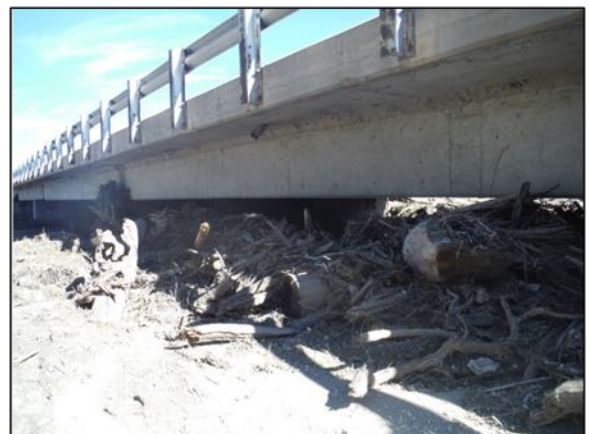
C-17-B over South Platte River – Debris accumulation up to low girder
