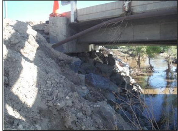
C-17-C over Little Thompson River – Right abutment scour
