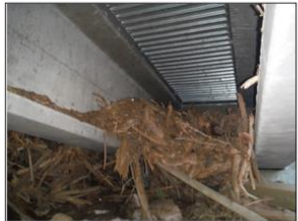
C-16-DK over Little Thompson River – Debris accumulation above low girder
