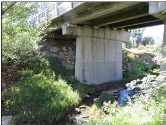
C-17-CZ over Draw –Bridge outlet showing steep gradient and channel downcutting
