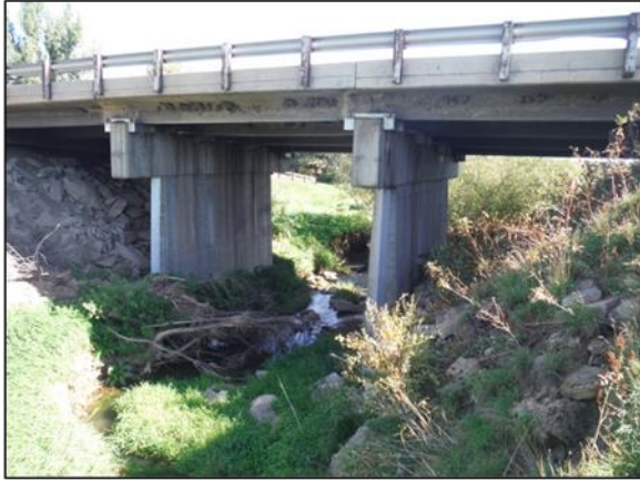
C-17-CZ over Draw – Center bay experienced several feet of channel downcutting
