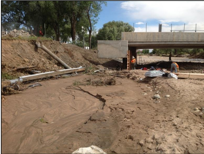
Failed right abutment on HW 36 at Lyons
