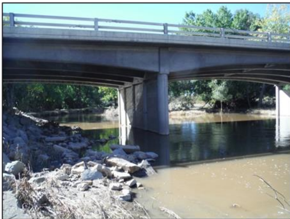
C-17-BL over Big Thompson River – Riprap loss at right abutment
