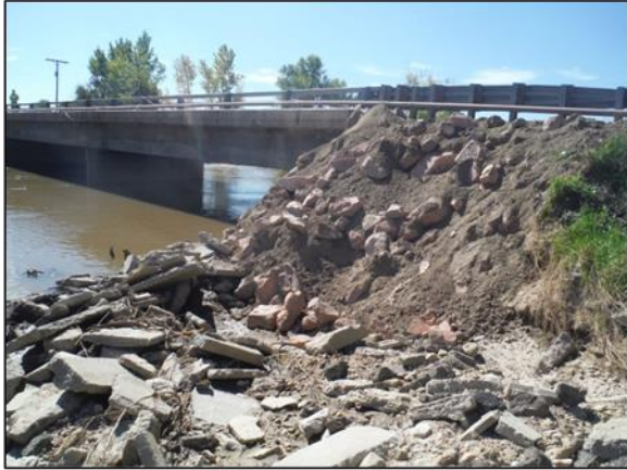
C-17-Z over Big Thompson River –Downstream left abutment scour
