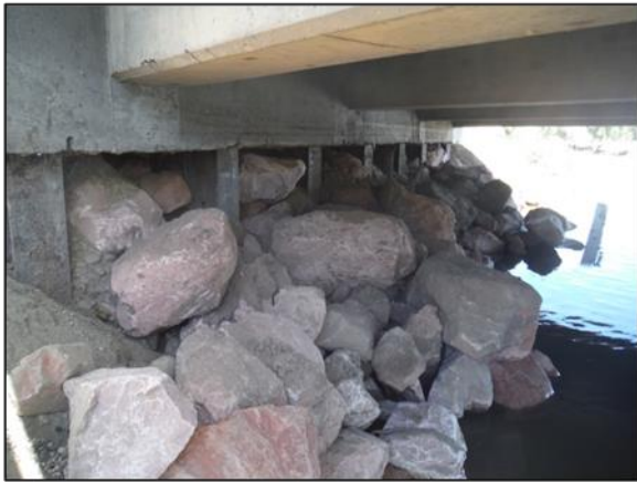
C-17-Z over Big Thompson River – Exposed left abutment piles
