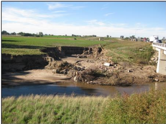
C-17-N over Little Thompson River – Channel and left embankment scour upstream of bridge
