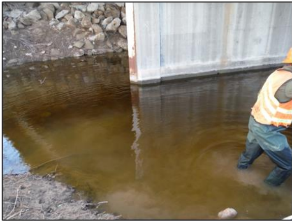
A-17-AC over Lone Tree Creek – Scour hole at left pier
