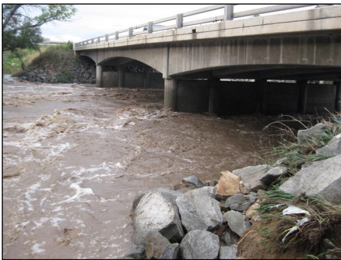
Big Thompson River at I-25, failed right abutment
