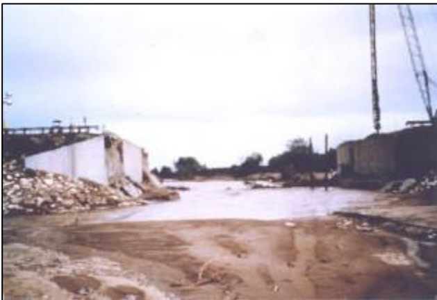
Figure 2. View of the failed bridge from the channel facing downstream. Note the failed left abutment.
