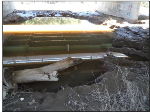
C-18-AG over South Platte River – Scour hole in between piers
