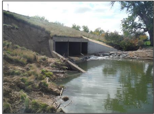
E-16-BC over Coal Creek – Significant scour hole downstream and from right abutment up to roadway
