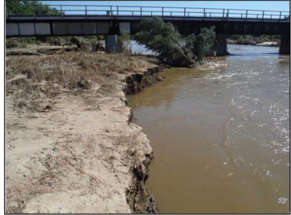
C-18-AG over South Platte River – Channel bank scour
