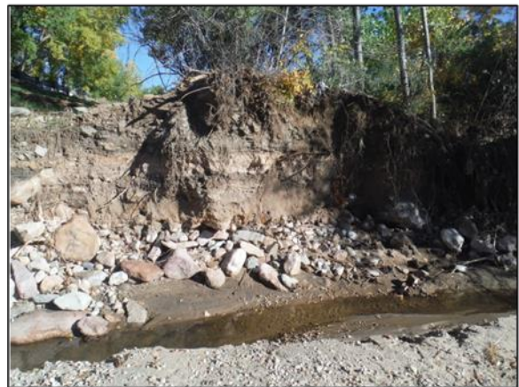
D-15-X over Left Hand Creek – Downstream embankment and channel failure due to contraction scour
