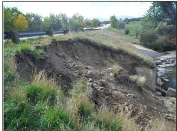
E-16-BC over Coal Creek – Scour hole from downstream right abutment to roadway
