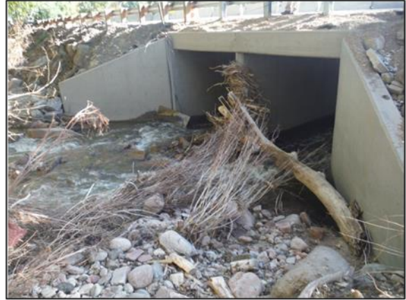
D-15-X over Left Hand Creek – Culvert inlet with debris and cobble accumulation
