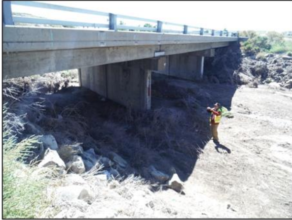
A-17-AC over Lone Tree Creek – Abutment riprap loss
