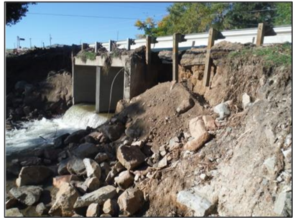
D-15-X over Left Hand Creek – Culvert outlet and abutment s show significant scour and undermining
