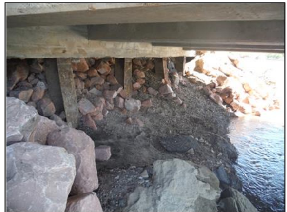
C-17-B over South Platte River – Exposed left abutment piles
