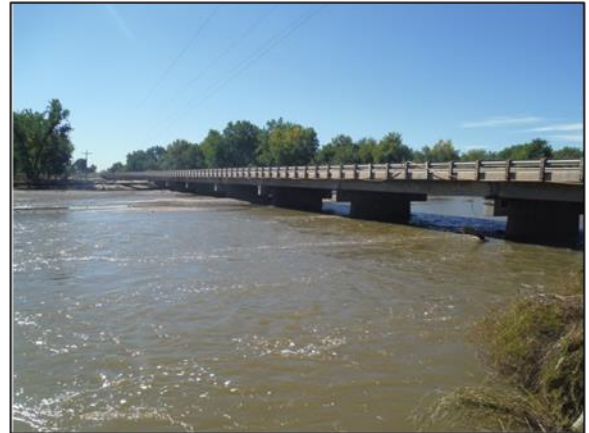
C-17-B over South Platte River – High flows and sediment discharges have changed channel morphology
