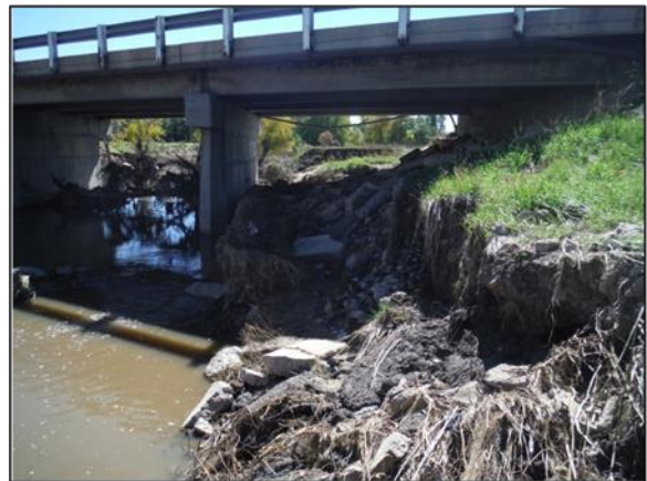
C-17-C over Little Thompson River – Left abutment and embankment scour downstream
