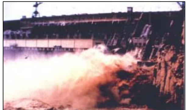
Figure 3. Sediment-flushing operation through Sanmenxia dam releases up to 90% of solids.
