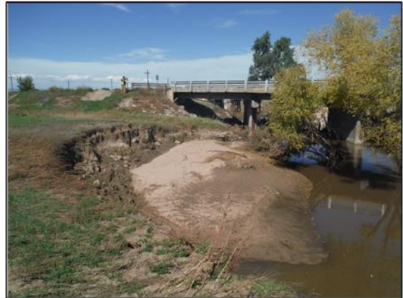
C-17-C over Little Thompson River – Channel and embankment scour leading to left abutment
