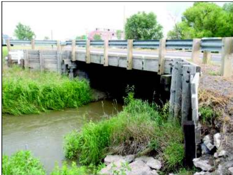
Figure 2. Bridge A-27-N over the Lodgepole Creek
