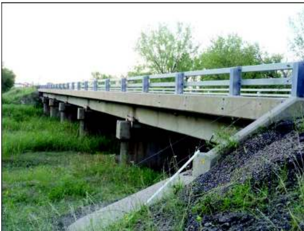
Figure 2. Bridge A-28-N over the South Platte River
