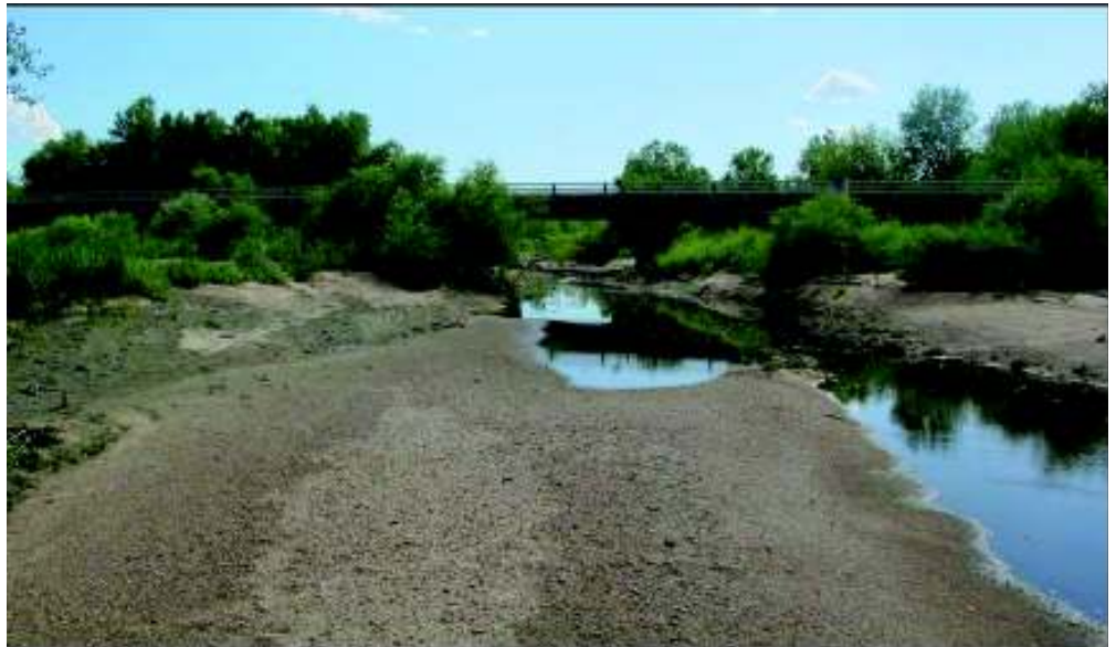
Figure 1. Bridge A-28-O over the South Platte River
