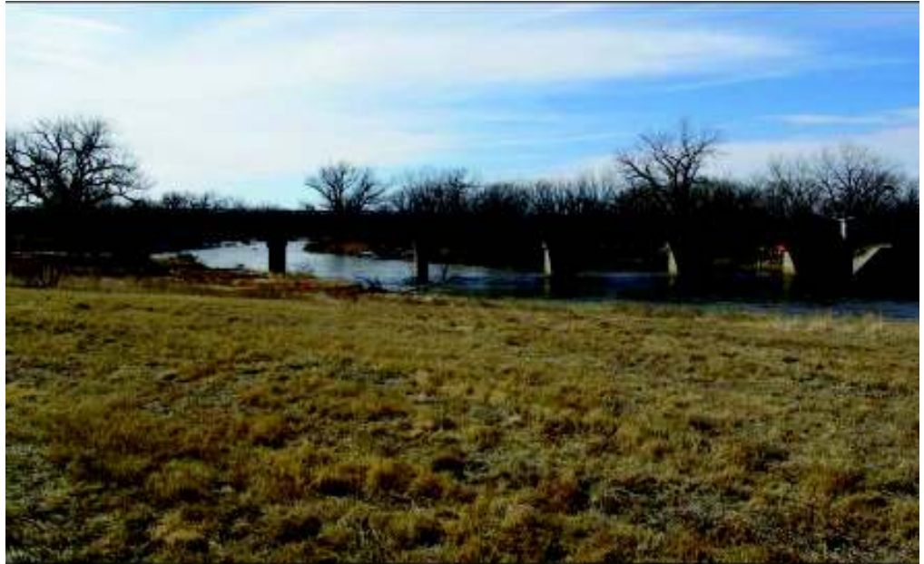
Figure 1. Bridge A-28-P over the South Platte River
