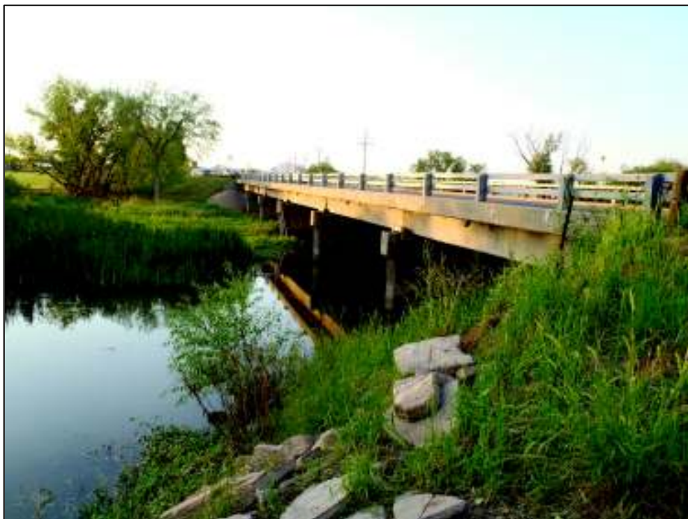
Figure 2. Bridge A-28-M over the South Platte River
