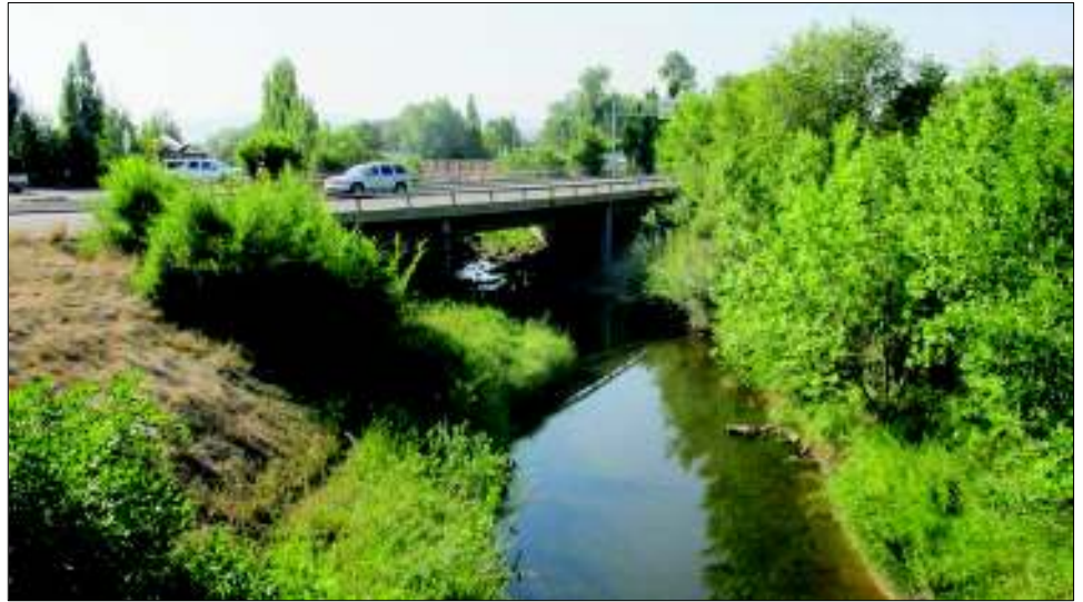
Figure 1. Bridge B-06-S over Fortification Creek
