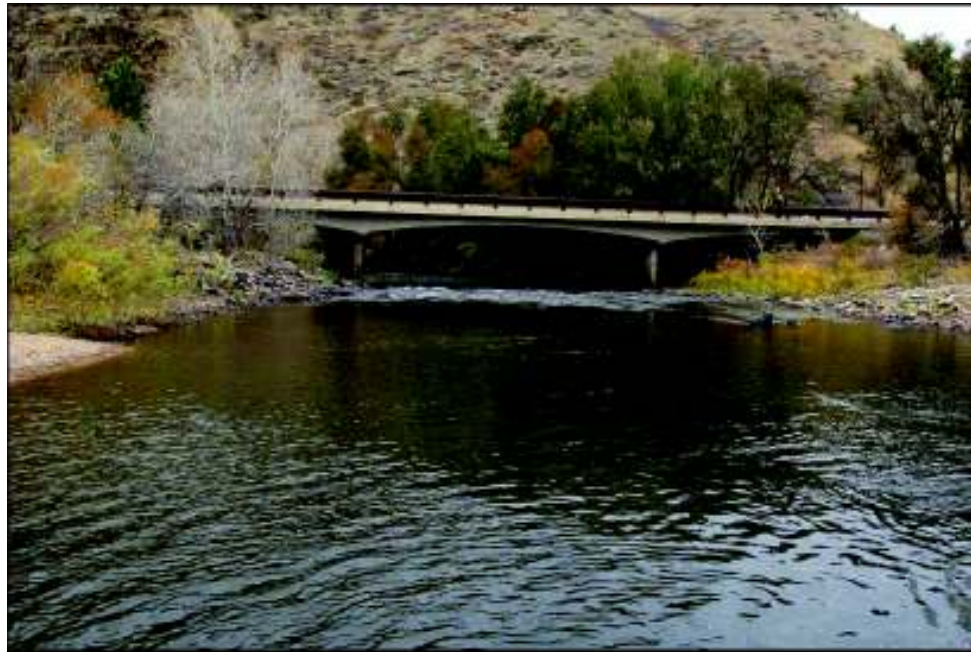
Figure 2. Bridge B-16-FT over the Cache La Poudre
