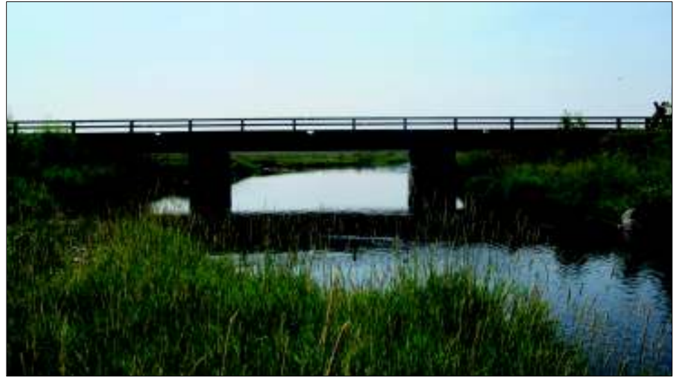
Figure 1. Bridge C-09-AR over Yampa River
