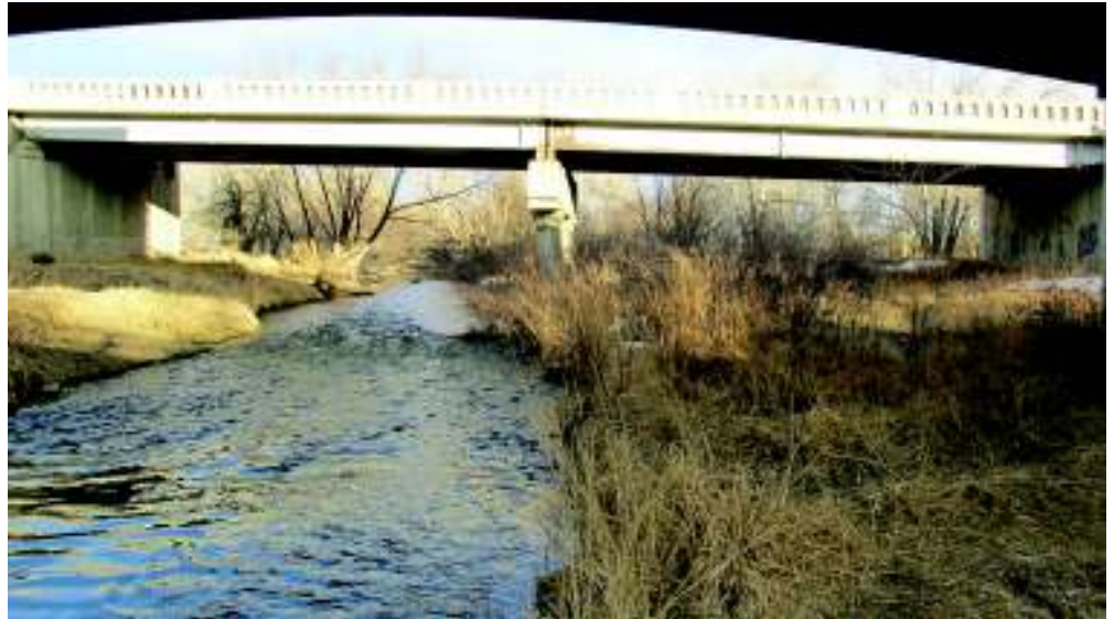
Figure 1. Bridge C-17-F over the Big Thompson River
