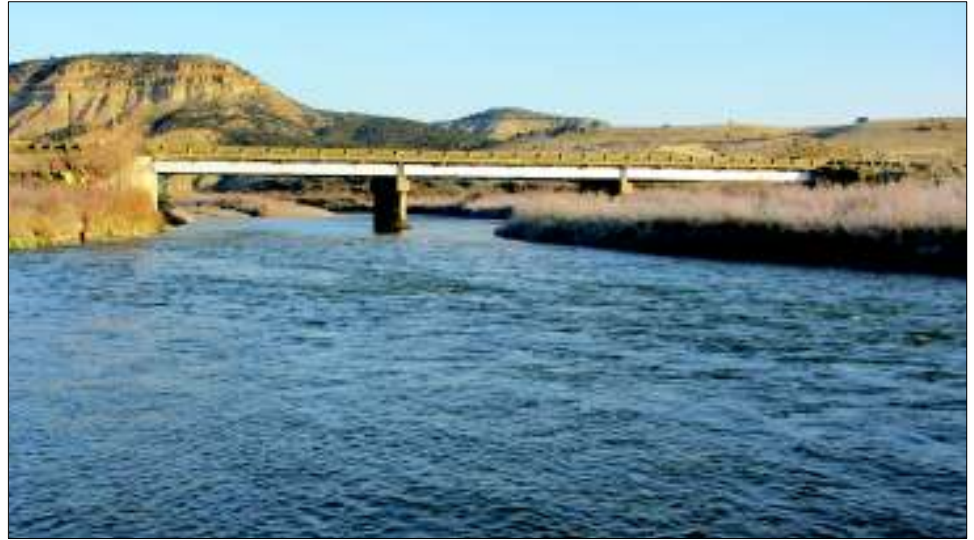
Figure 1. Bridge D-03-A over the White River
