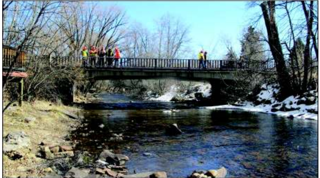
Figure 2. Bridge D-15-A over the North St. Vrain Creek
