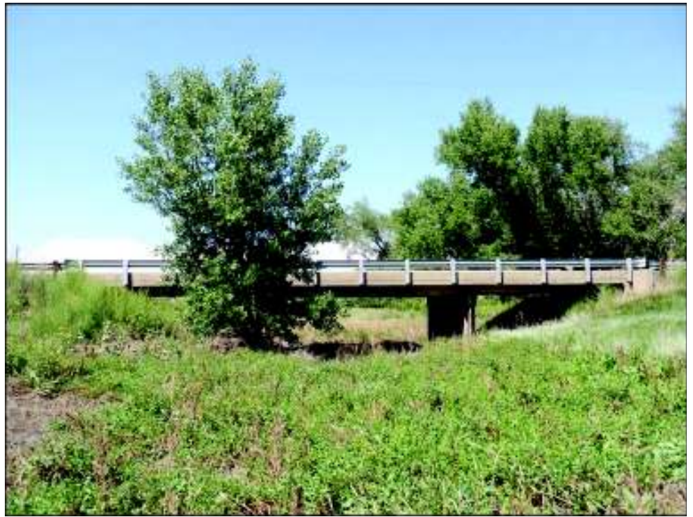
Figure 2. Bridge D-20-T over the Colorado River
