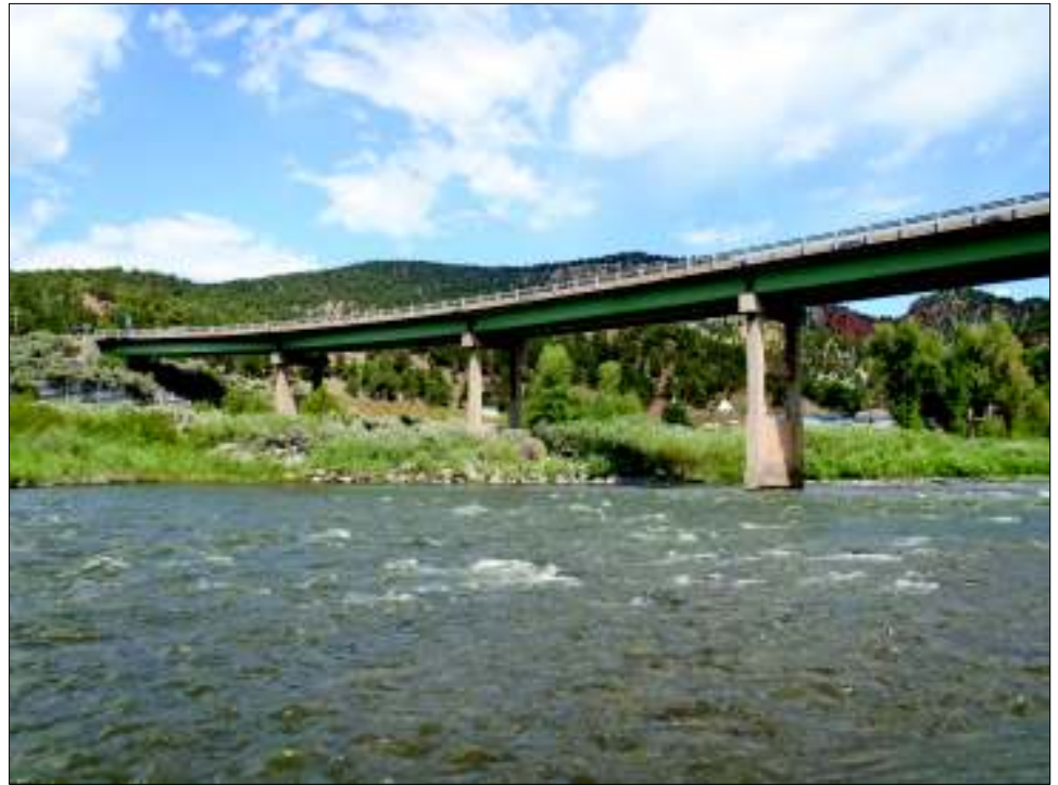
Figure 1. Bridge E-10-A over the Colorado River
