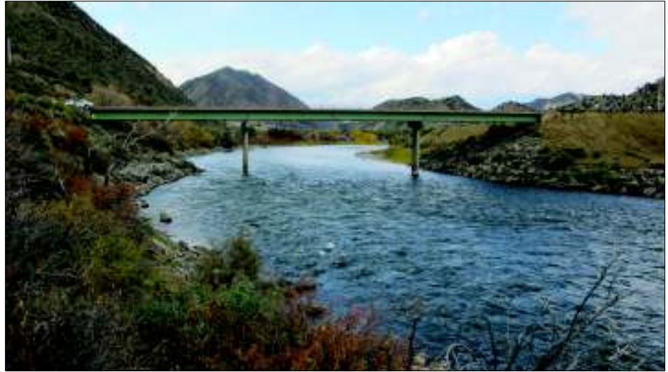
Figure 1. Bridge F-06-M over the Colorado River
