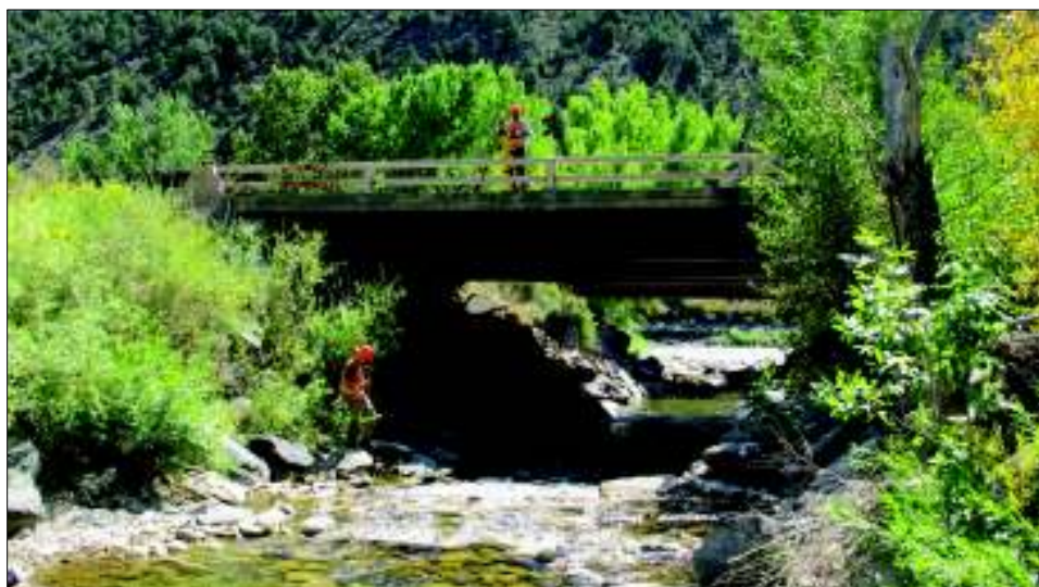
Figure 1. Bridges F-06-O and F-06-P over Elk Creek
