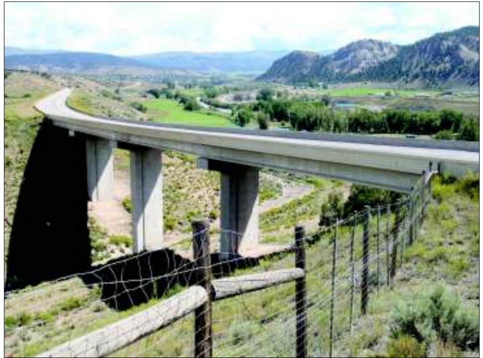
Figure 1. Bridge F-09-AF over Cottonwood Creek
