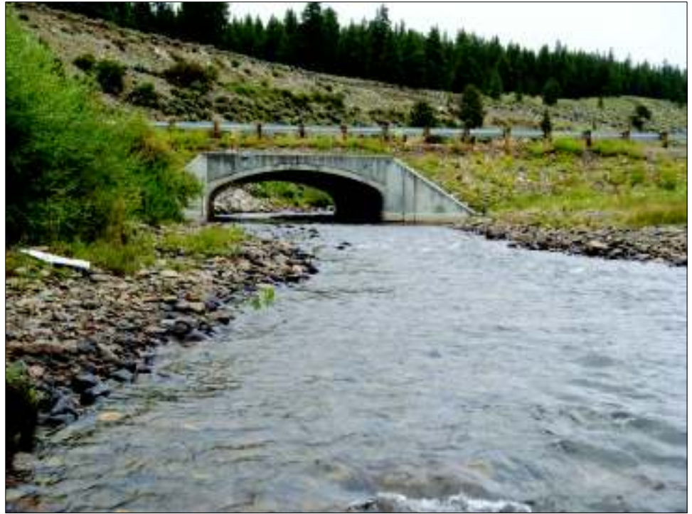
Figure 1. Bridge G-11-C over the East Fork Arkansas River
