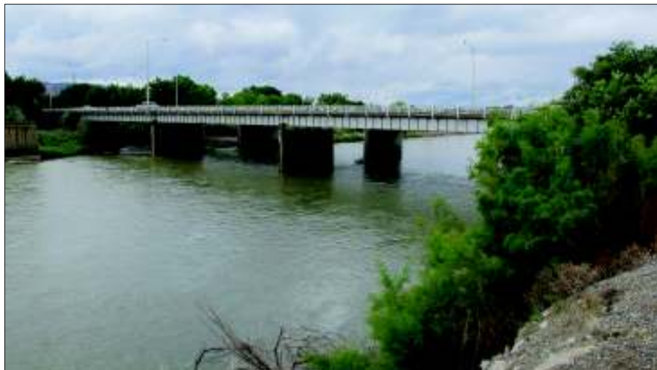
Figure 1. Bridge H-02-GC and H-02-S over the Colorado River
