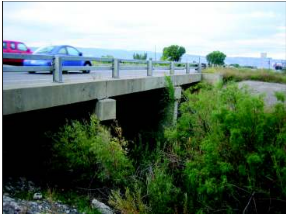
Figure 1. Bridge H-03-Z over Lewis Wash
