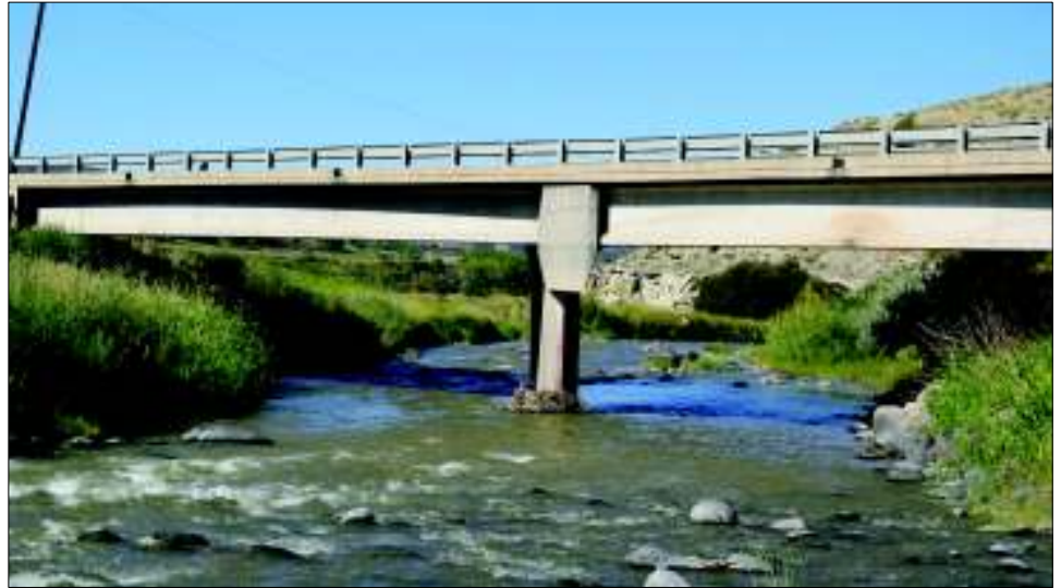
Figure 1. Bridge H-04-S over Plateau Creek
