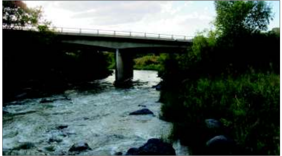
Figure 1. Bridge H-04-Z over Plateau Creek
