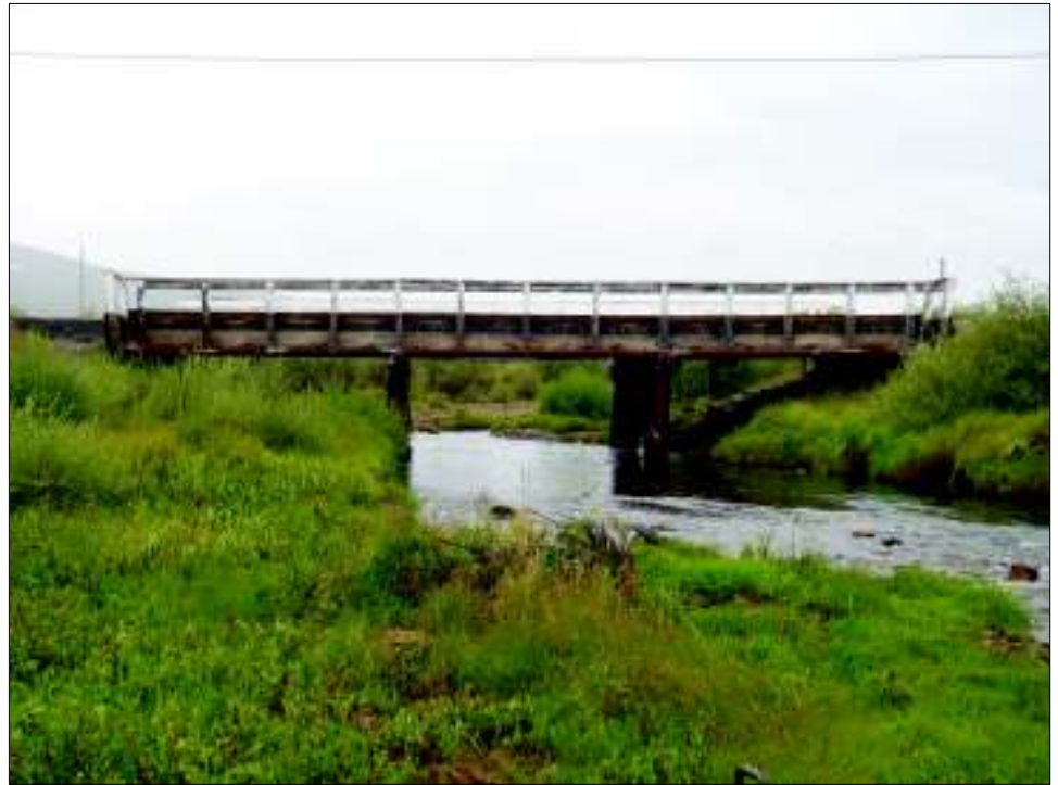
Figure 1. Bridge H-11-U over Lake Fork Creek
