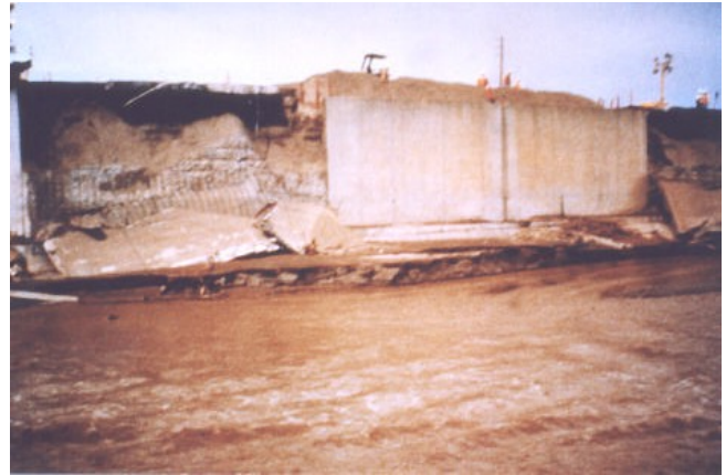
Figure 3. View of the failed bridge from the channel facing downstream. Note the failed left abutment.
