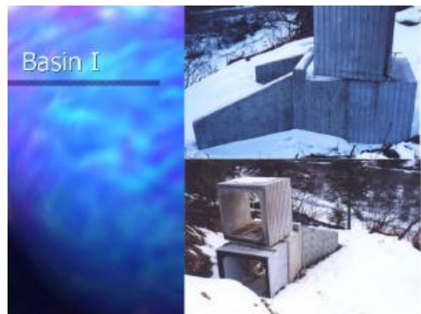
Figure 9. Culvert outlet and pre-fabricated culvert sections.
