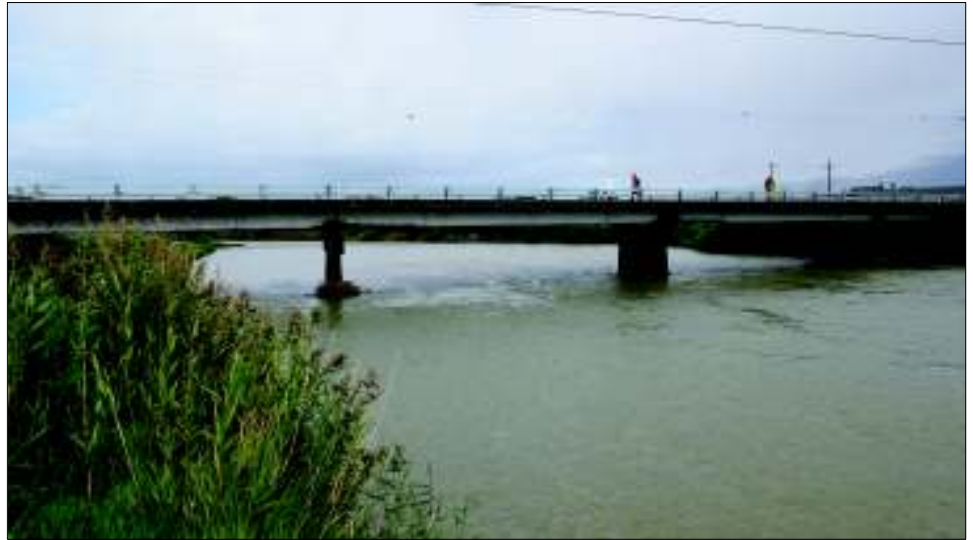
Figure 1. Bridge I-03-A over the Gunnison River
