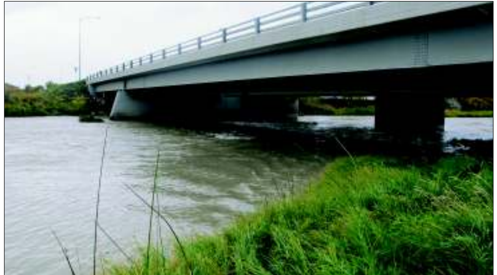
Figure 1. Bridge I-04-K over the Gunnison River
