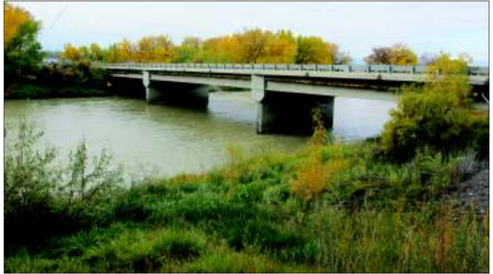
Figure 2. Bridge I-04-M over the Gunnison River
