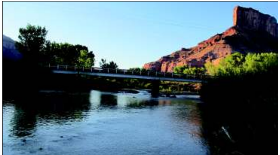
Figure 1. Bridge J-01-C over the Dolores River
