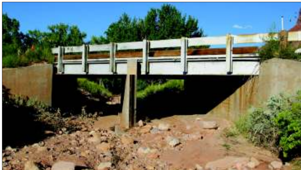
Figure 1. Bridge J-01-D over John Brown Creek
